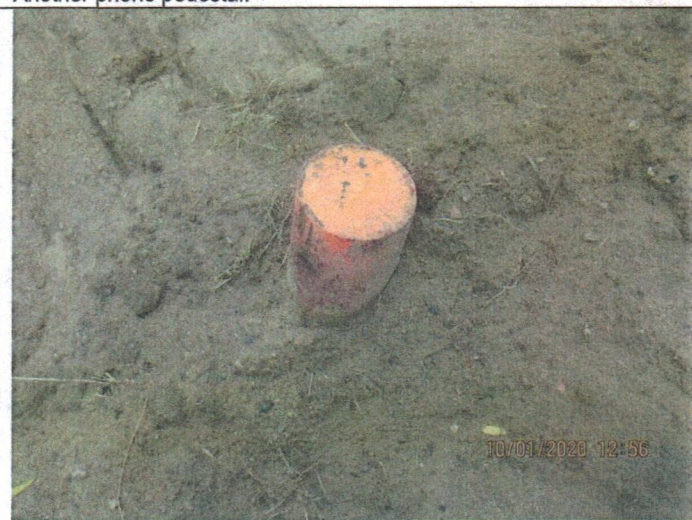
Pipe – possible cleanout.
