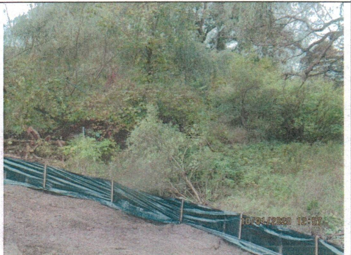
Existing crossover of gully toward Roll Drive.
