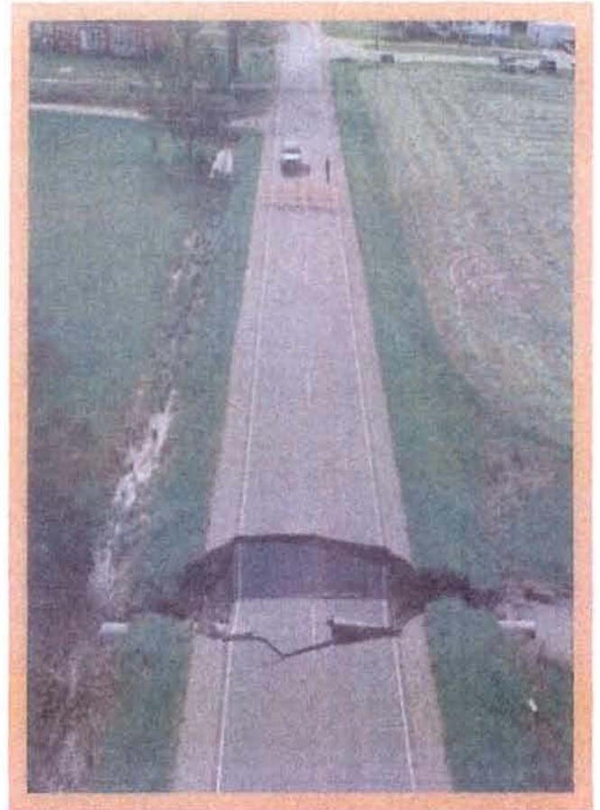
Road damage from storm
