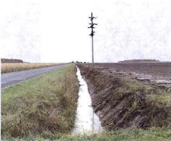
Bierlein Drain – Denmark Township
