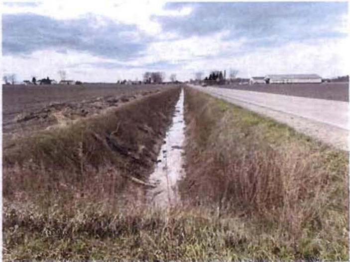
Curry Improvement Drain – Akron Township
