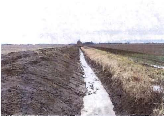
Carlton Intercounty Drain – Columbia/Elmwood Township with Huron County
