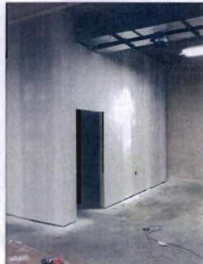
Drywall on new divider walls, at the new facility
