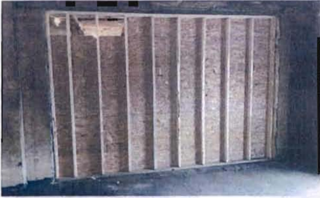
New wall construction, in the new facility
