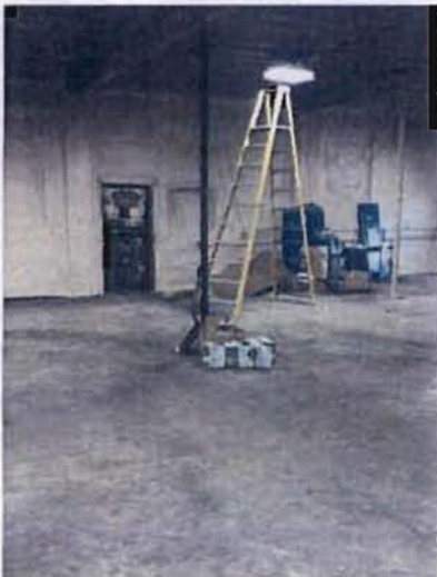
Painting the ceilings, at the new facility
